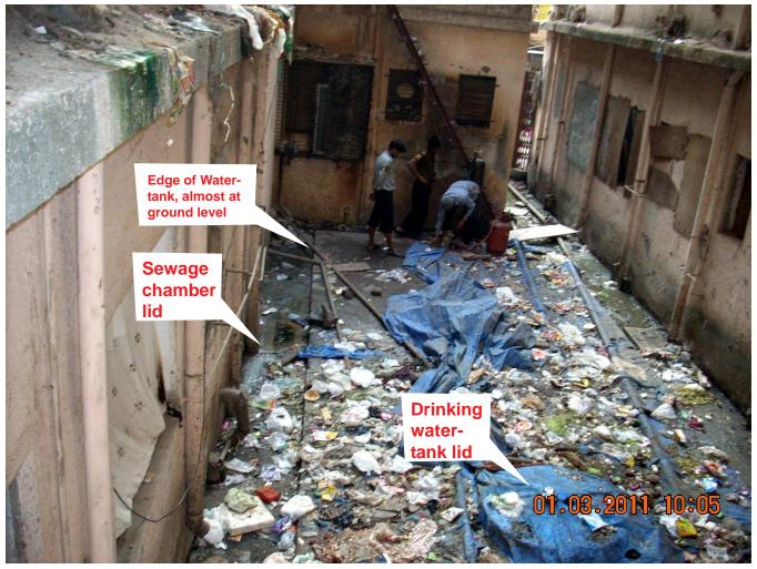
Underneath this layer of filth is the water-tank and the sewage chamber, side-by-side. There is a rule that the sewage chamber should be 1.5 metres from the building, so that the foundations are not eroded. There are rules and regulations that water supply and sewage chamber must be kept apart, and that water-supply tank must be substantially above ground level. As you can see, all these rules have been overlooked by both RNA Corp and MMRDA..
